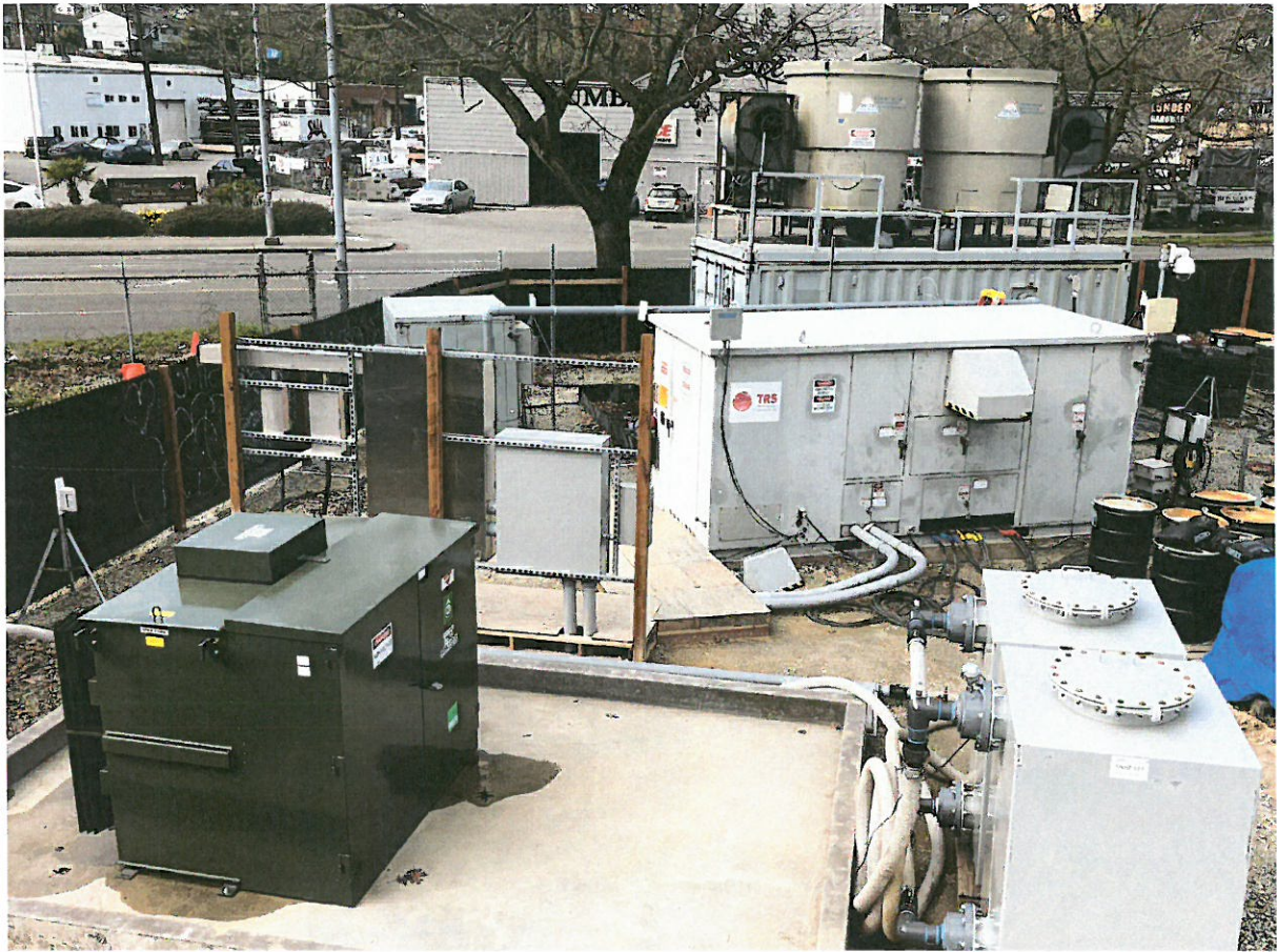
Typical ERH equipment compound. The equipment located in the center background are the condenser/cooling towers. The unit is 20' long by 8' wide by approximately 16' high. The equipment located in the center is the ERH power control unit (PCU). The PCU for this site will be 15' long by 8' wide by 9' high.
