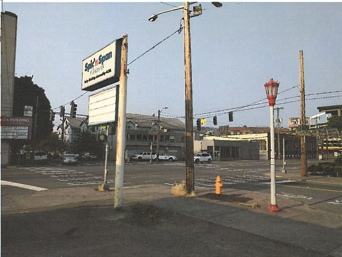
Right-of-way facing southwest
