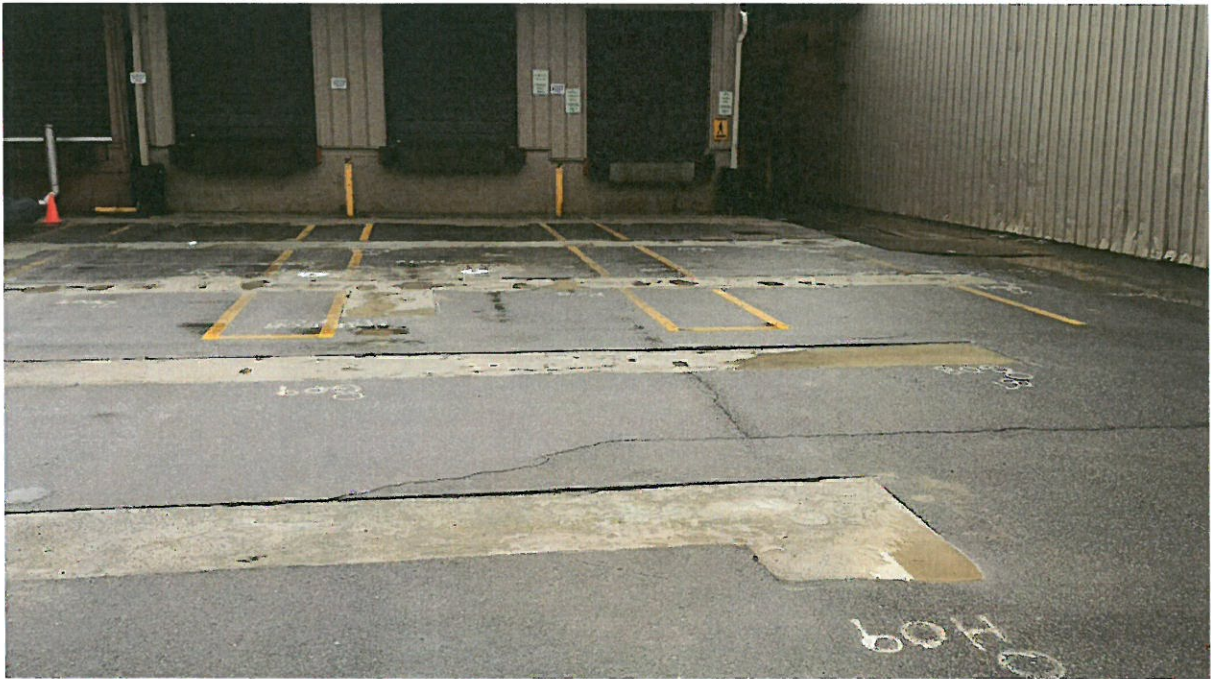
Trench in parking lot repaired with controlled density fill (CDF) during ERH operations. The CDF is removed and replaced with asphalt at the completion of operations.
