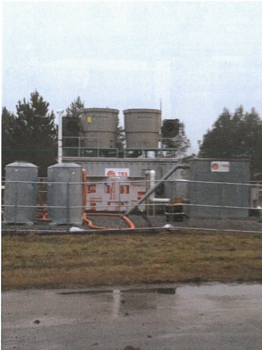
ERH equipment compound without privacy screening on fence. Vapor phase granular activated carbon vessels and discharge stack are located in the foreground.
